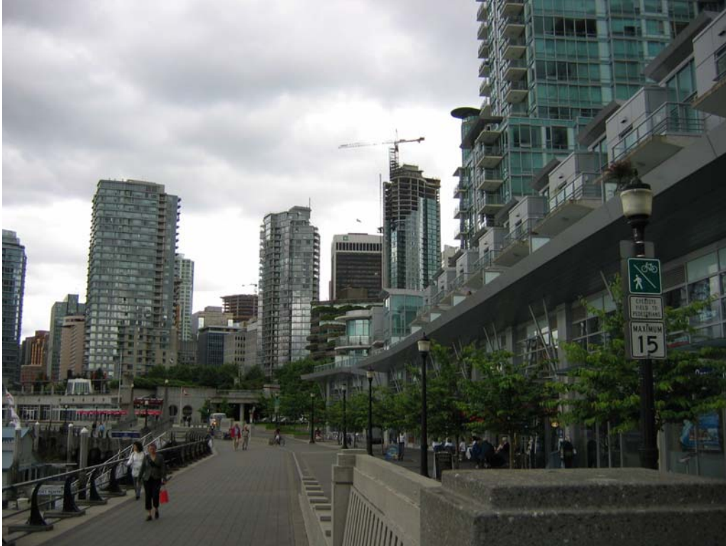
Figure 2. Vancouver has become well known for its slender towers with bases that address the street, containing a mix of residential and commercial uses.
