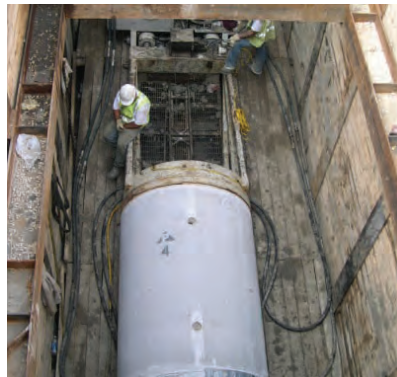
Akkerman Jacking System Source: AECOM
