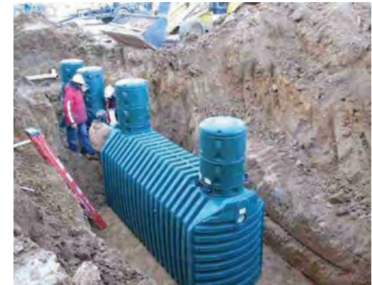
Source: Brac Systems Rainwater Harvesting
