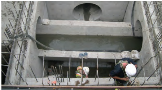
Weir Overflow, King and Logan Source: AECOM
