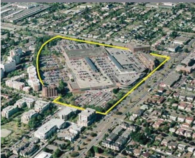
Existing Oakridge Centre mall adjacent to the Canada Line in the Oakridge Municipal Town Centre is an important opportunity site.
