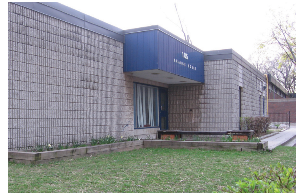
Existing Community Centre at 105 Grange Court
