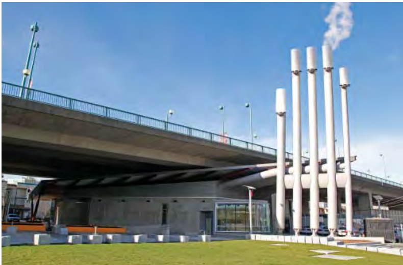
Neighbourhood energy utility building at South East False Creek, Vancouver
