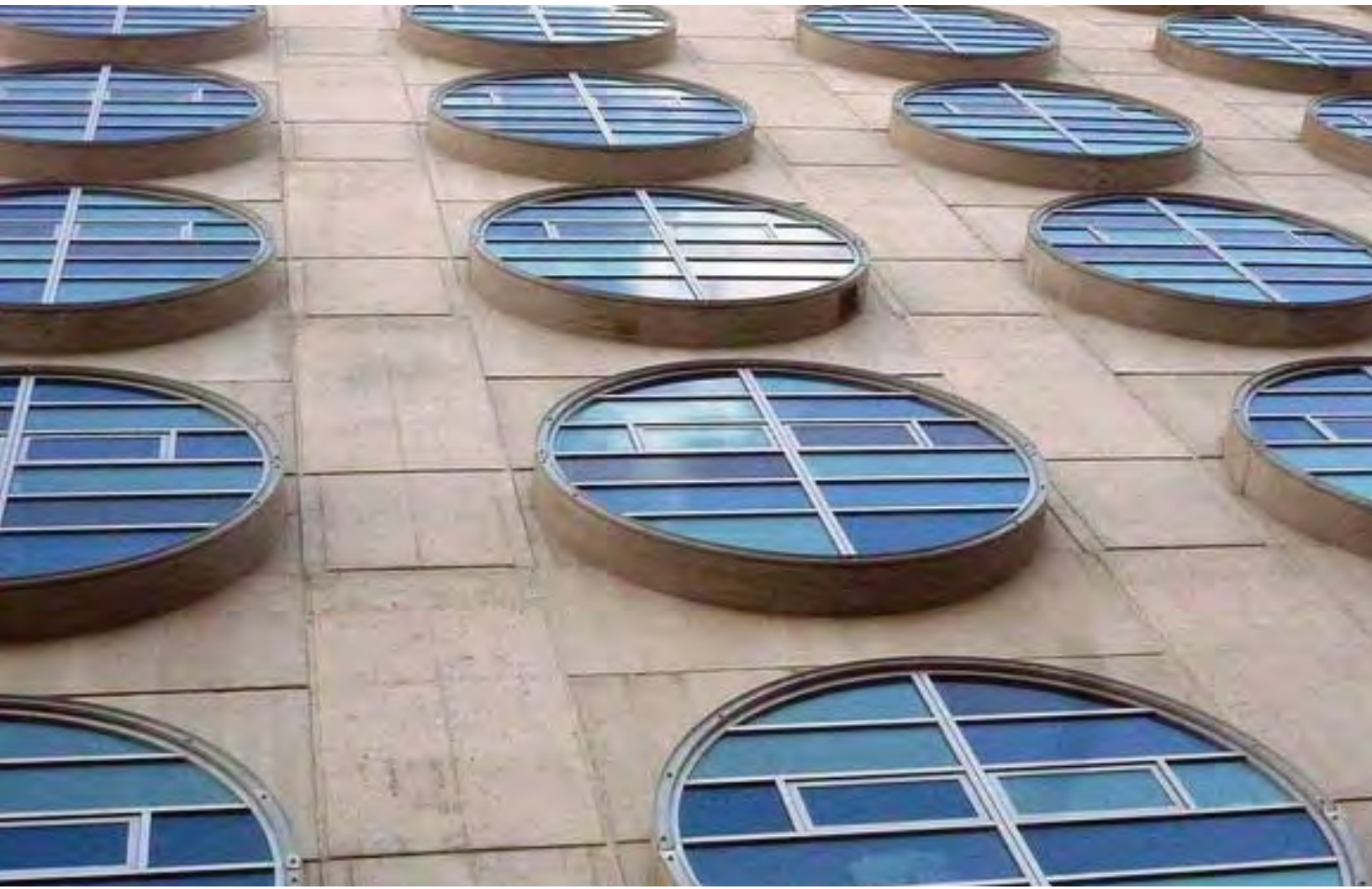
BC Cancer Research Center, first LEED Gold health care facility in Canada. Includes heat recovery system to offset ~60% of heating load, energy-efficient lighting and operable windows to maximize natural light and improve indoor air quality.
