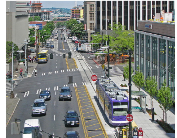
Dedicated transit infrastructure incorporated into the street
