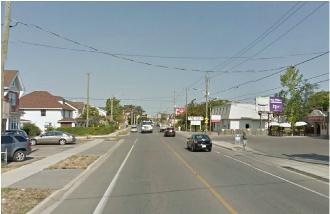
Regional Road 81 facing west
