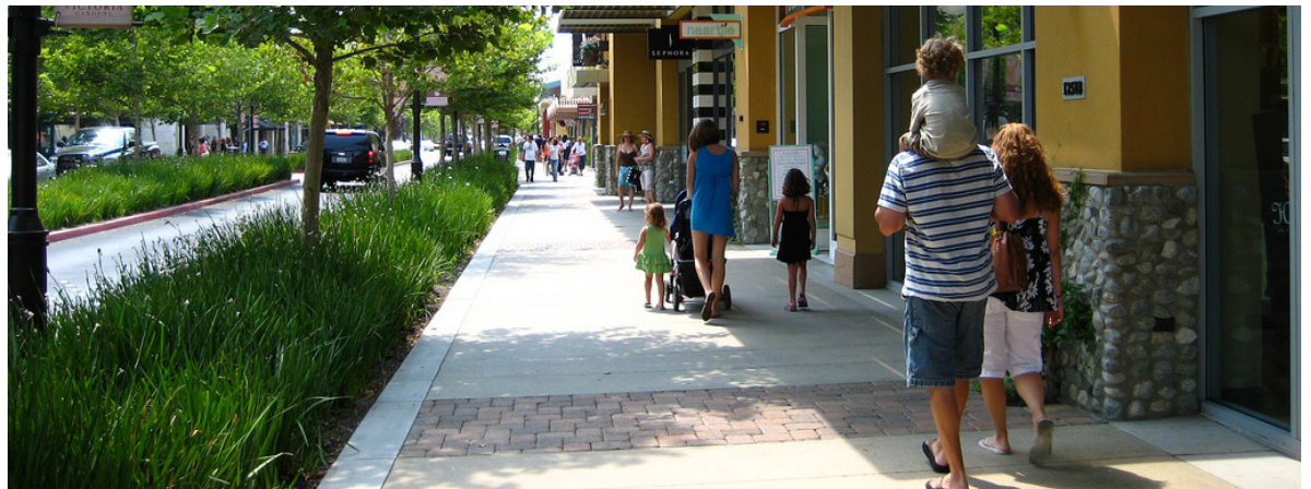
Wider sidewalks can accommodate planting and street furniture and improve the pedestrian experience
