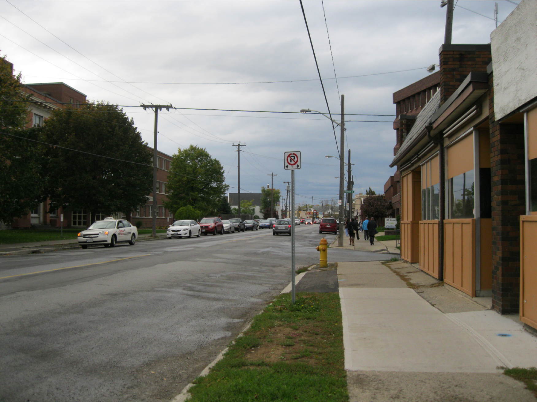
● Site 1: Existing condition
