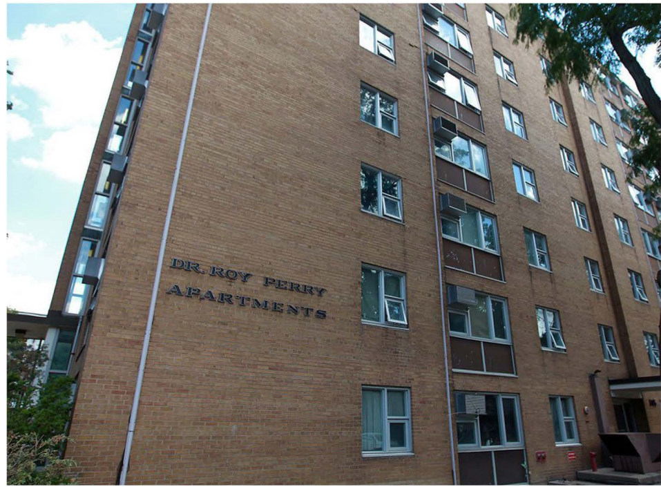
Figure 11. Dr. Roy Perry Apartments exterior (Source: Google, 2022). Retrieved May, 2012.
