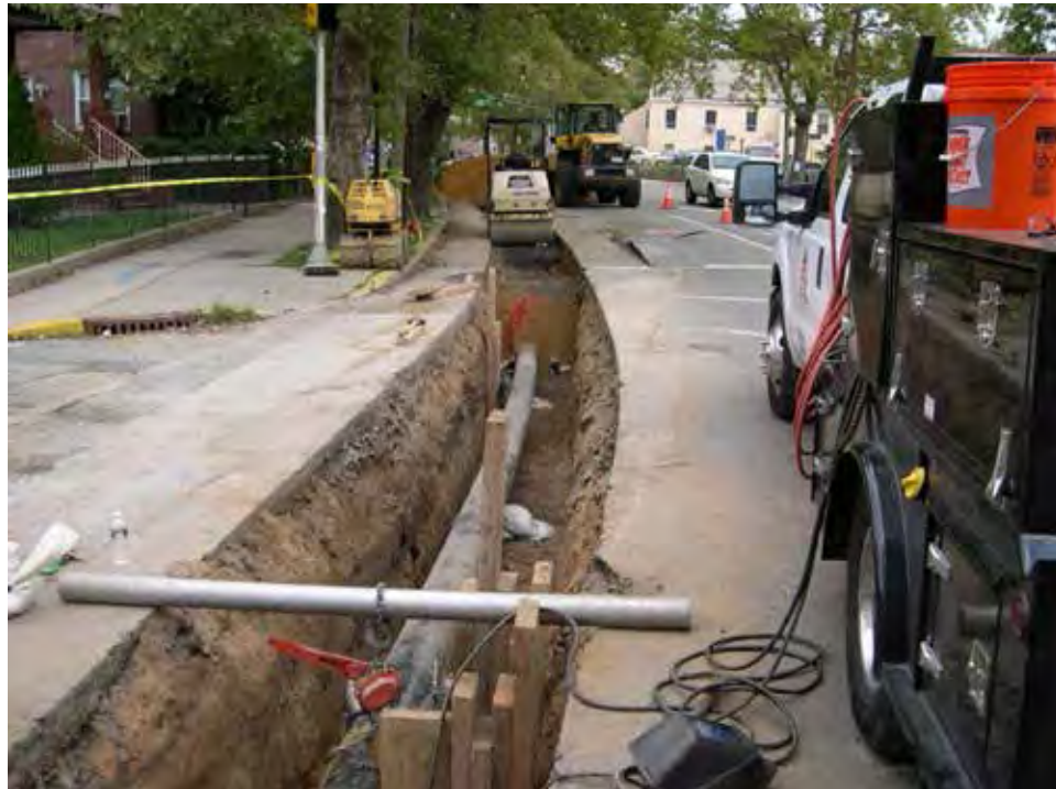
Image showing construction work to bury transmission lines
