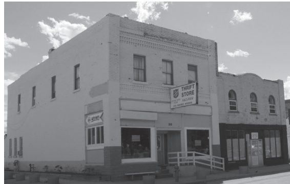
Buildings as it looks today
