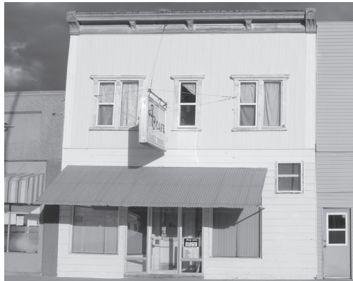
Buildings as it looks today
