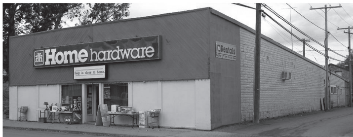
Buildings as it looks today
