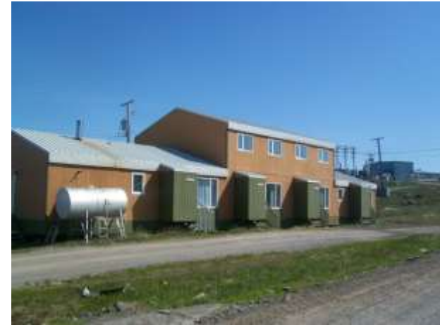
A multi-unit residential building (ca. 1980s) with compact rectangular design (minimal structural projections into yards) and protection against wind and snow.
