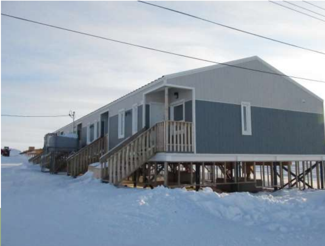
Five-plex residential building in Kugluktuk, built on piles drilled into bedrock.
