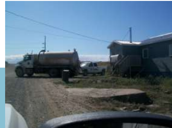
Trucked water, wastewater, and fuel services. (A few communities also have utilidor.)
