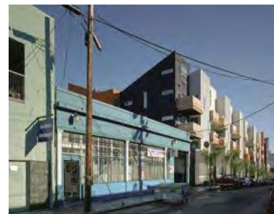
Neighborhood street that has developed and evolved overtime as needs change while remaining a vital part of the community
