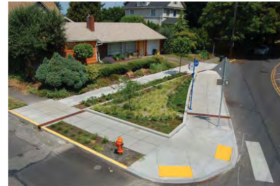
Street park at street corner
