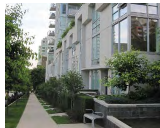
This residential development transitions from individual private patios to a semi-private planting zone to the public sidewalk
