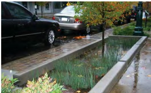
An example of sustainable stormwater retention techniques within a street tree planting bed
