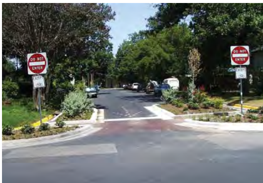
Example of a curb extension shortening the distance needed for a pedestrian to cross the street.
