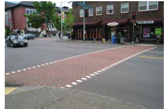
Example of a marked crosswalk
