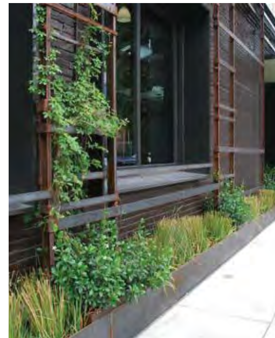
Example of sustainability practices such as stormwater retention and exterior shading incorporated into the design of a building
