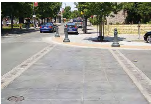
Curb extension and enhanced crosswalk materials increase safety of pedestrians
