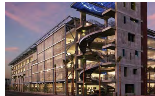
Examples of Parking Structures that exhibit the same principles for good building design
