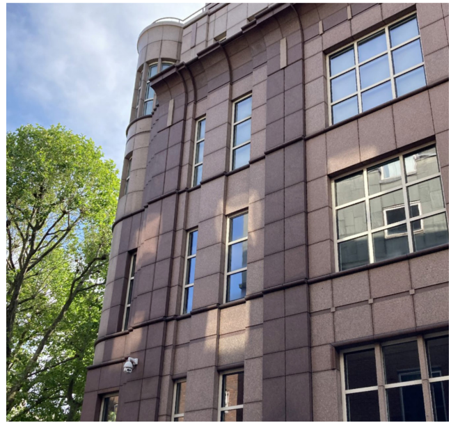
Figure 1.7. Ha/f developed a reuse strategy for Waterhouse Square's granite facade, in collaboration with Local Works Studio, London. By prioritizing deconstruction, on-site reuse, and low-carbon fabrication, the project reduces waste and emissions while advancing the goals of London's Circular Economy Roadmap for sustainable building practices.
